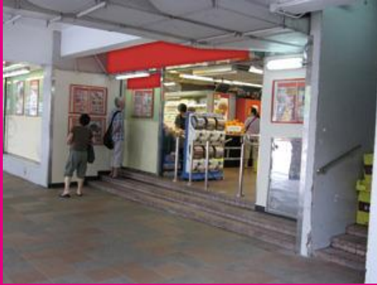
Example of Barriers: Stepped entrance
